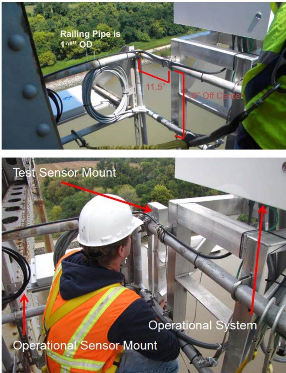
Figure 19. Sensor mounting.
