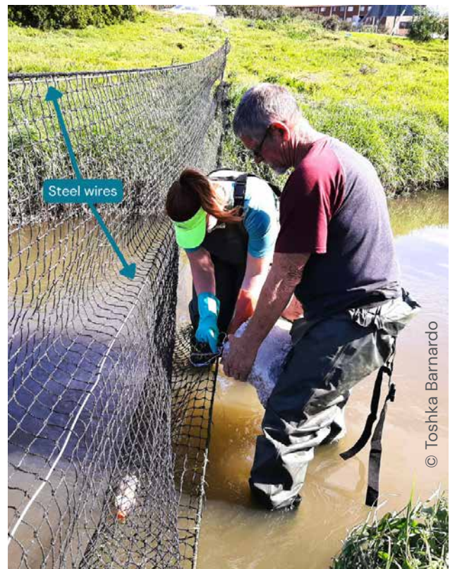
Figure 7: The bottom of a litter net in Gqeberha, South Africa, is secured with concrete blocks. Note that the net is reinforced with wire at the top and in the middle.
