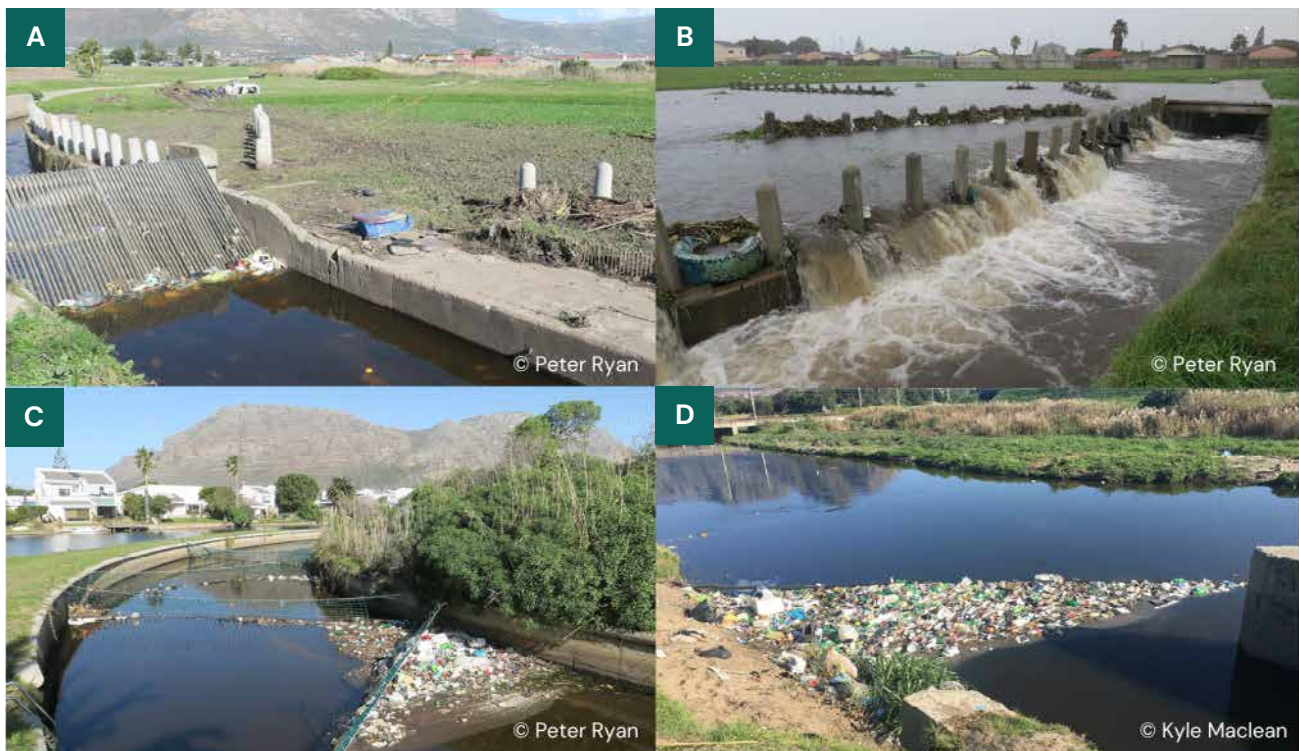
Figure 2: Examples of low-tech devices used to collect litter in waterbodies. (A) An inclined grid screen installed by the City of Cape Town municipality on a canalised section of a river in Cape Town, South Africa. This system works well under low- to moderate-flow conditions if serviced regularly. However, it may rapidly become blocked during high-flow conditions, requiring an overflow basin with bollards (B) to trap larger debris items. (C) A series of nets with increasingly finer mesh installed by an NGO in Zandvlei, Cape Town. (D) Litter boom installed by The Litterboom Project (an NPO) on the Black River, Cape Town.
