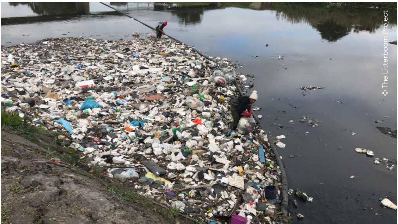
Figure 10: By placing the boom/net at a 45–60° angle, litter is directed to one side of the waterway, reducing drag force on the trap and making it easier to clean.
