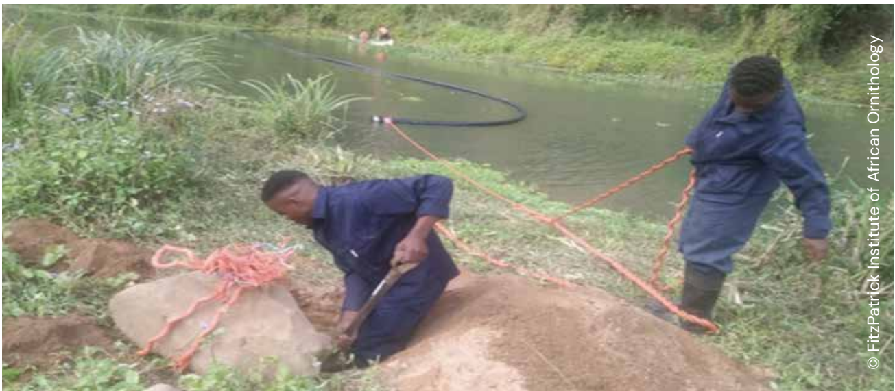
Figure 11: Workers anchoring a litter boom by attaching it to a boulder, to be buried in the bank above the floodline.
