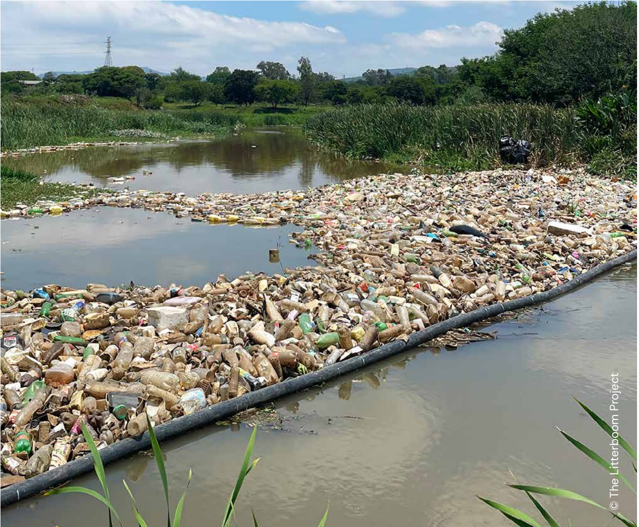
Figure 4: An HDPE pipe boom installed by The Litterboom Project in South Africa.
